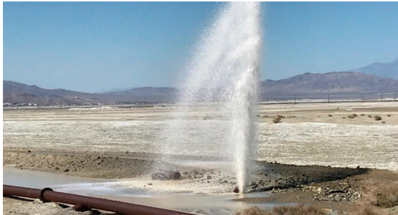
The earthquake damaged a pipe. Source: Accuweather.com
