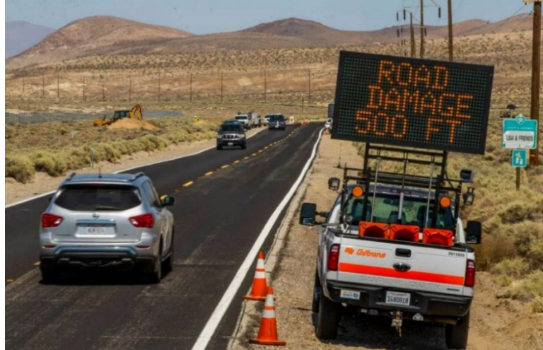
Caltrans crews repairing Highway 178. Source: Reviewjournal.com
