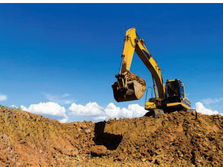
Figure 6. Image of bulldozer removing soil from a pit.
